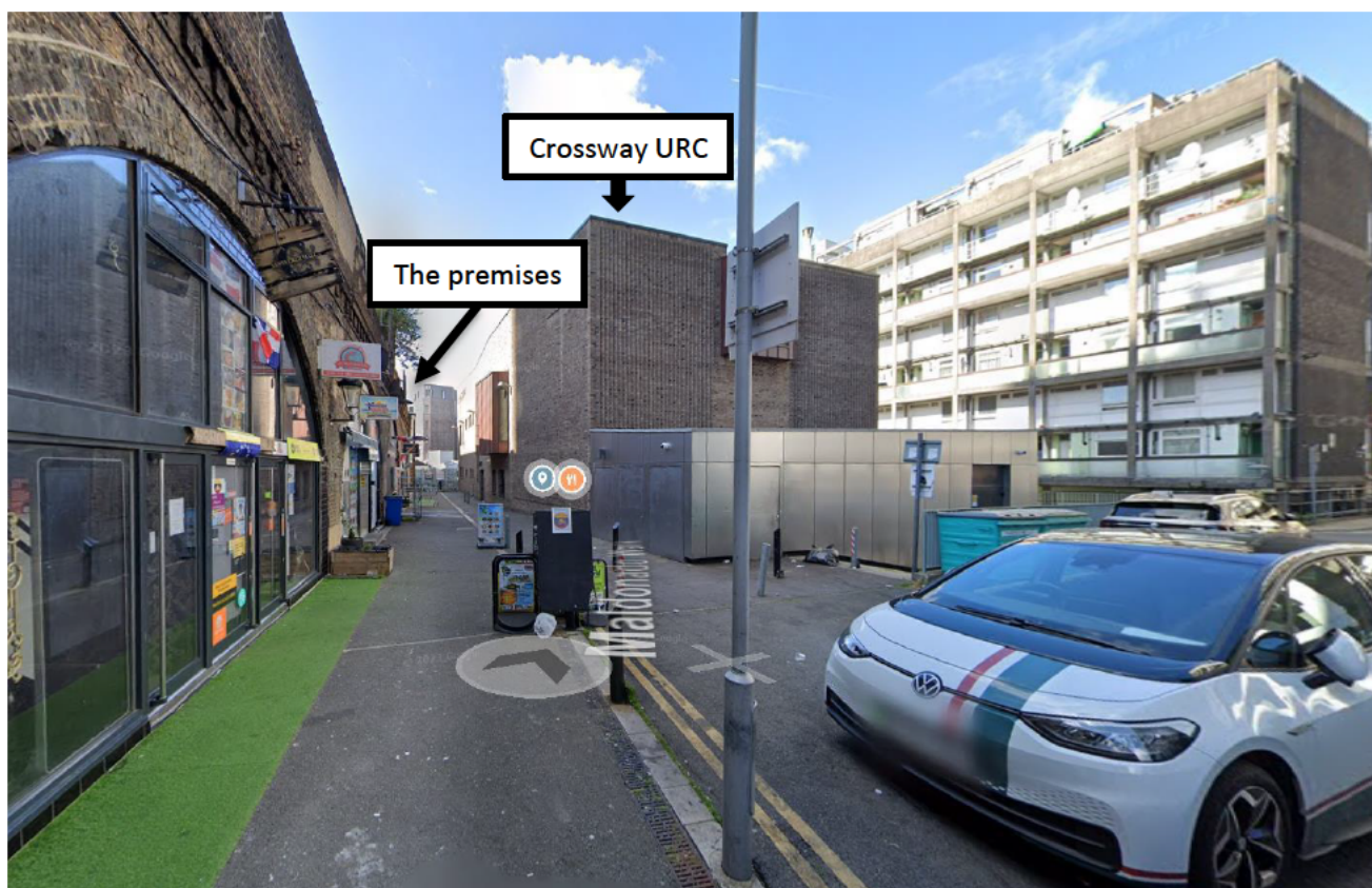
Figure 5: View looking south down Maldonado Walk showing Crossway United Reformed Church
